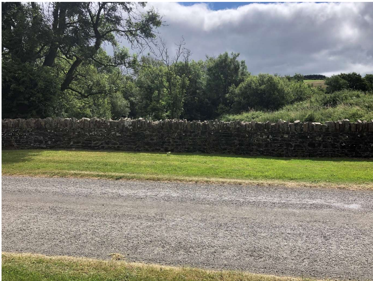
Photo 15-20: Stone walls and other stonework
